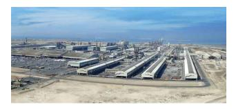
EGA's Al Taweelah site is located in Khalifa Industrial Zone Abu Dhabi. It includes an aluminium smelter, a casthouse, a plant that manufactures carbon anodes and the head office. We also have desalination plant that meets our water needs and a power plant to generate electricity. This consists of nine gas turbines and four steam turbines with a generation capacity of 3,100 megawatts.
